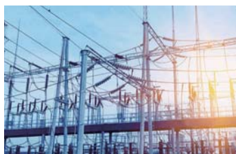
Power Generating Companies
